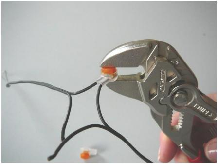
4. Press - watch the wires don't slip off the holes.
